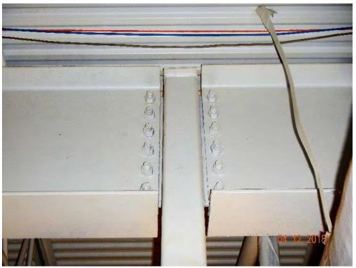
Photograph 3 – Unbraced top of column in equipment room
