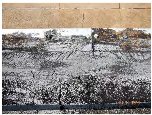
Photograph 5 – Modified bitumen membrane on Field House roof
