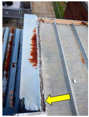
Photograph 8 – Deterioration where metal seam roof is adjoined to coping flashing
