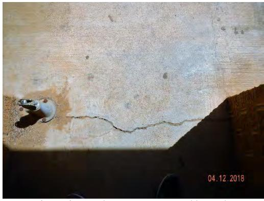
**Photograph 28** – Cracking at gymnasium exterior slab-on-grade
