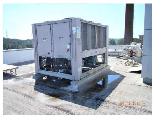
**Photograph 20** – Standing water underneath roof top unit at press box
