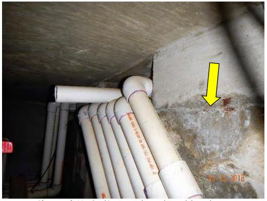
Photograph 11 – Cracking at crawl space beneath hot tub area
