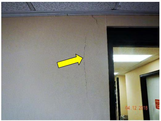
Photograph 7 – Cracking at the interior wall of the Field House addition
