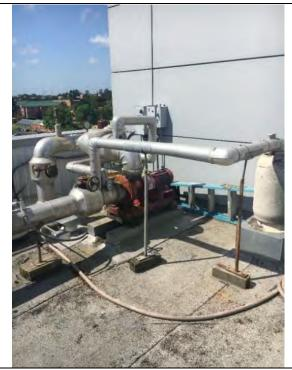
Football Stadium: Air cooled chiller's chilled water pump. Needs redundant pump. Loss of pump shuts down AC in Press Box.
