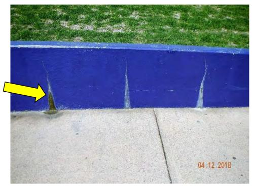
Photograph 15 – Leaks at cracks in walkway retaining wall
