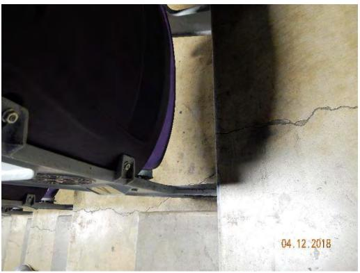
Photograph 21 – Cracking at the coliseum seating
