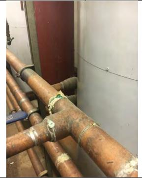
Field House: Domestic water hot water piping needs to be replaced – Pict 2
