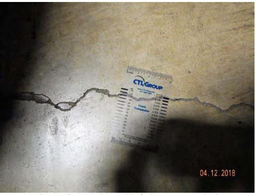
**Photograph 24** – Cracking at slab of coliseum concourse level
