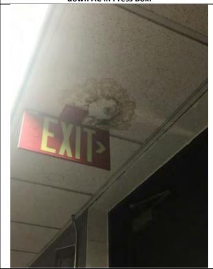
Coliseum: Condensate leaks from chilled water insulation above ceiling - Pict 1
