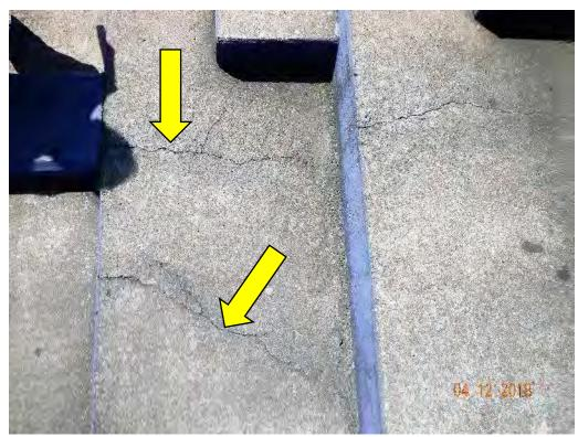
Photograph 13 – Typical cracks at grandstand treads and risers
