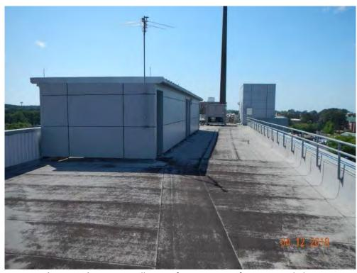
**Photograph 18** – Overall view of Press Box roof; note granule loss
