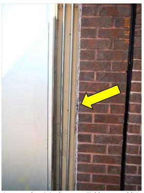
Photograph 9 – Deterioration at sealant joint between Field House addition and original Field House
