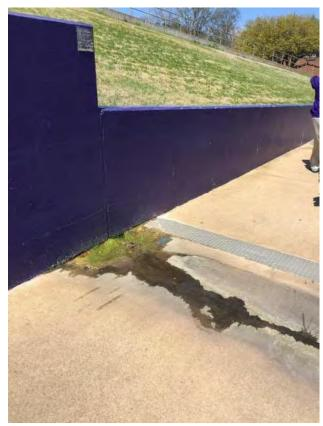
**Photograph 16** – Leaks at cracks in walkway retaining wall and steel plate over crack/spall in walkway
