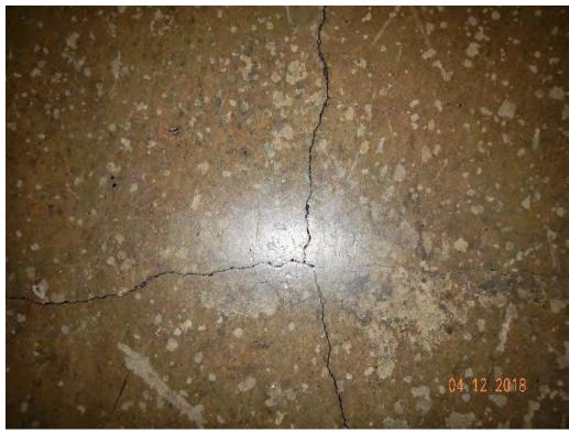
**Photograph 23** – Cracking at slab of coliseum concourse level
