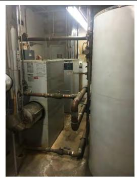
Field House: Domestic Water Boilers and associated piping needs to be replaced - Pict 1
