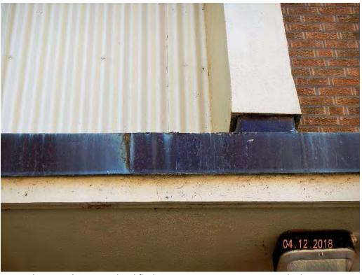
**Photograph 32** – Oxidized flashing at gymnasium exterior north elevation
