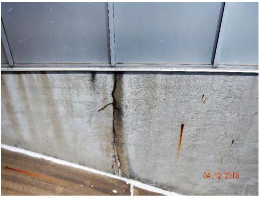
Photograph 10 – Leak at crack at south exterior elevation
