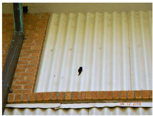
Photograph 31 – Hole at gymnasium exterior corrugated asbestos cement board
