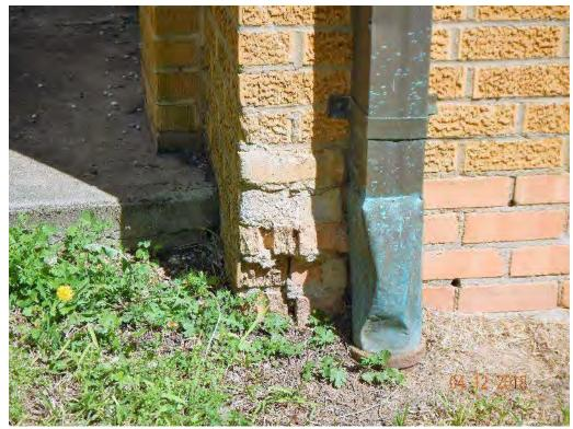
**Photograph 33** – Spall at bottom corner of gymnasium addition
