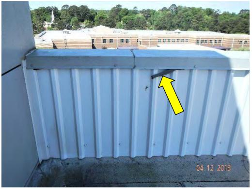
Photograph 19 – Detached foam closure material at metal coping
