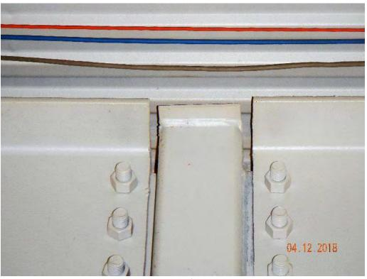
Photograph 4 – Unbraced top of column in equipment room
