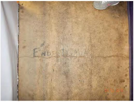
**Photograph 26** – Cracking at concrete at gymnasium seating level
