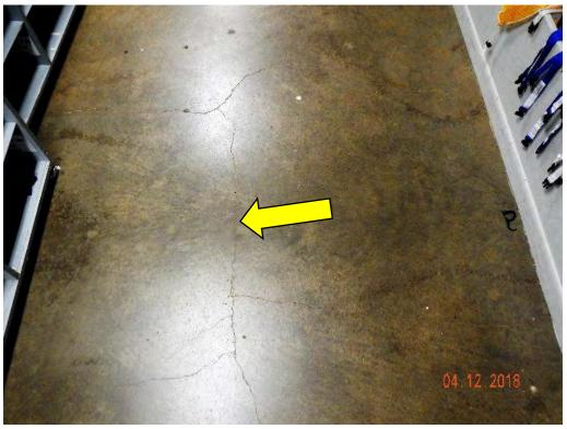
Photograph 2 – Cracking at slab on grade in Field House equipment room
