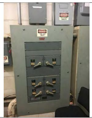
Field House: Original Fused/Switch Switchgear needs to be replaced.
