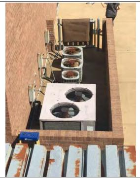
Field House grade mounted condensing units need to be replaced.
