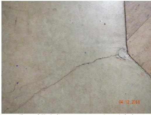
Photograph 27 – Cracking at concrete at gymnasium seating level
