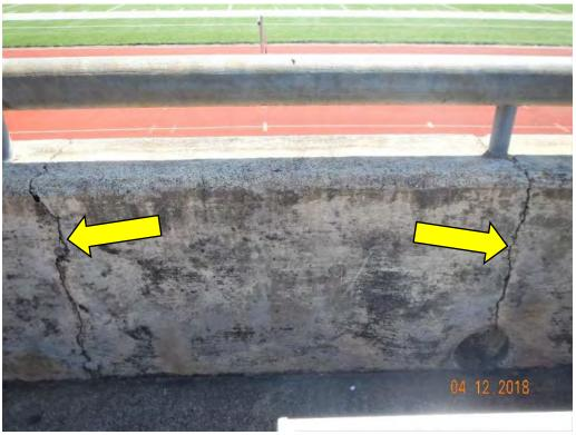
Photograph 14 – Cracks at walkway wall
