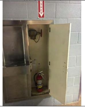
Coliseum: No sprinkler system. Only 4 dry standpipes served from FDCs on building exterior
