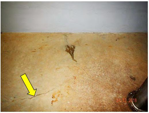
Photograph 6 – Cracking at slab on grade at lower level of Field House addition
