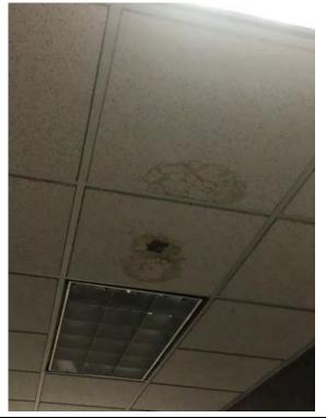
Coliseum: Condensate leaks from chilled water insulation above ceiling - Pict 2
