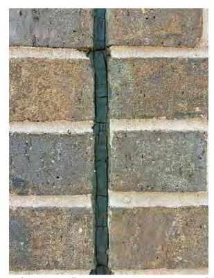
Photograph 34 – Control joint at Wellness Center exterior veneer in deteriorated condition
