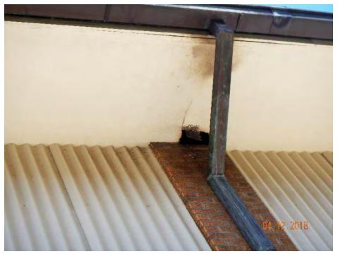
**Photograph 30** – Hole at exterior south elevation of eave at gymnasium
