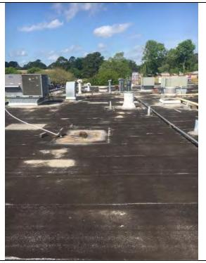
Field House Roof: No secondary roof drains installed
