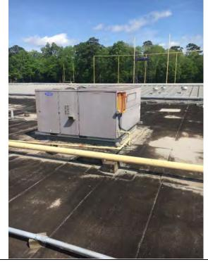
Field House Roof: RTUs need to be replaced.
