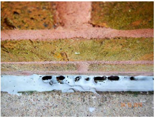
Photograph 12 – Deterioration of joint sealant at intersection of brick veneer with site paving
