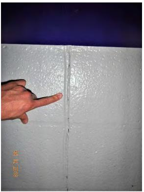
**Photograph 25** – Cracking at control joint at perimeter wall of coliseum
