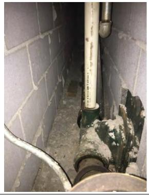
Coliseum: Plumbing Chase – Water Closet Carriers and sanitary piping needs to be replaced.
