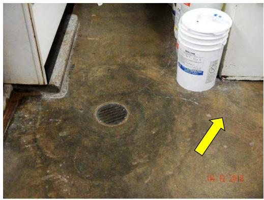
**Photograph 1** – Cracking at slab on grade in Field House laundry room
