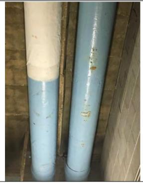
Coliseum: Chilled water piping needs to be replaced. It's original and beginning to get pin hole leaks.
