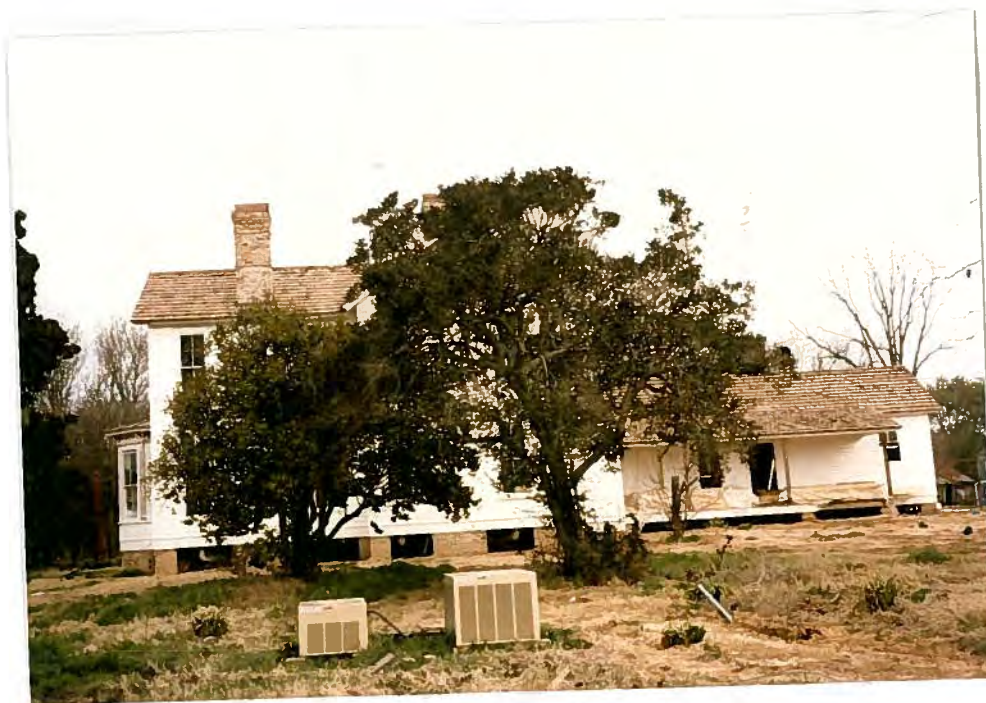
Above: Right Side From Front - South
