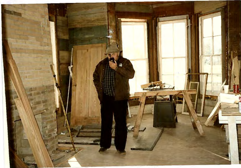
Owner, Samuel Floyd Vaughan III Inspects Restoration on the Interior
