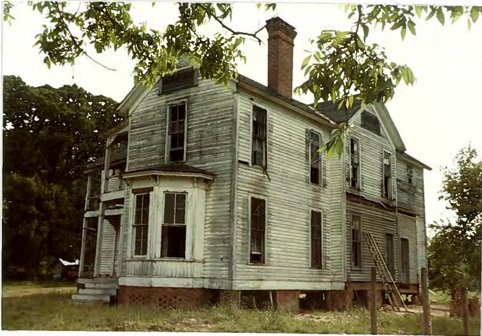
As the Restoration Gets Underway
