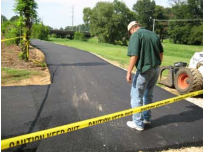
Dr. Creech tests out the new asphalt trails
