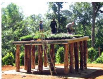
Planting the green roof pavilion at the Pineywoods Native Plant Center
