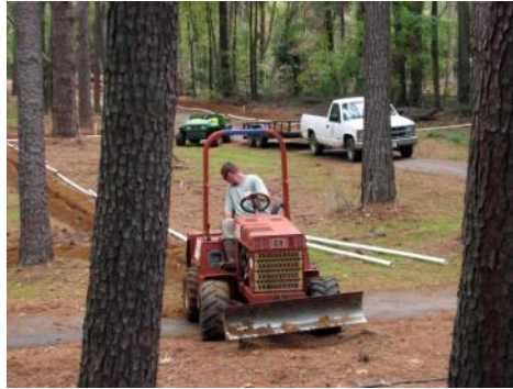
Brad Waguespack operates a ditch witch in the SFA Rec Trails and Gardens to create irrigation lines.
