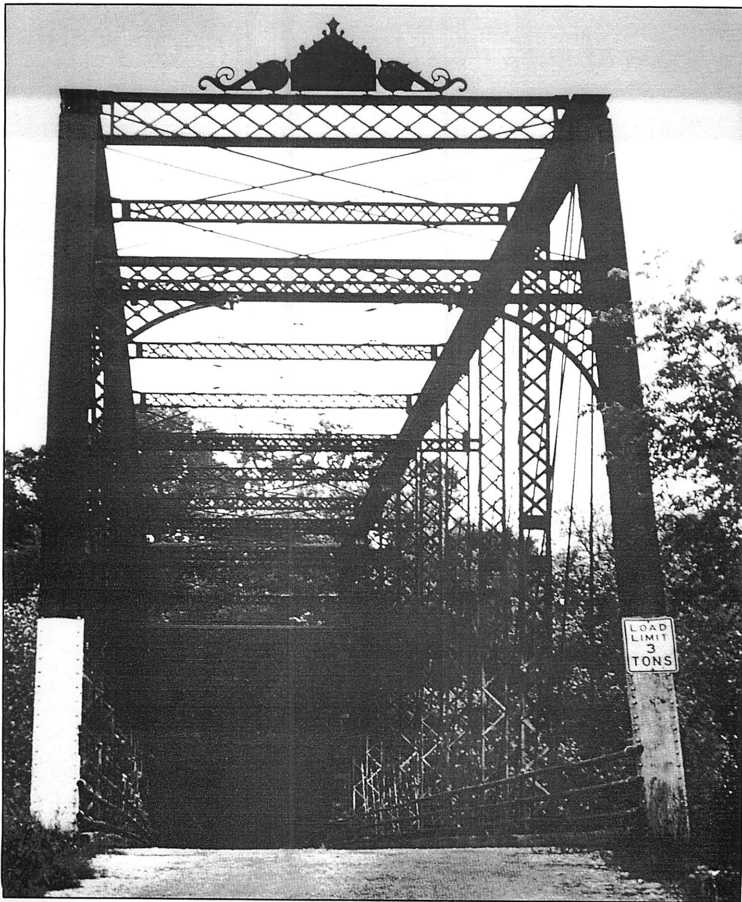
Old toll bridge on Old Highway 81 across the Lampasas River, between Belton and Salado in Bell County. This cast iron truss bridge was built in 1889.
