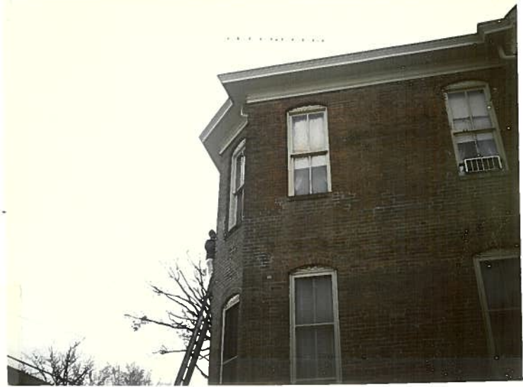
Kolak arch over window
