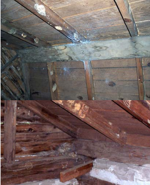
Figures 4.8, 9 and 10 show the extensive white rot along the interior of the roof. White rot can be seen on the sheathing, rafters and the partition walls of the second floor.
