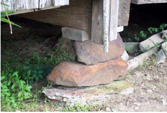
Figures 3.2 and 3.3 show another piece of wood in a precarious position and two red bricks support the weight of the house.
