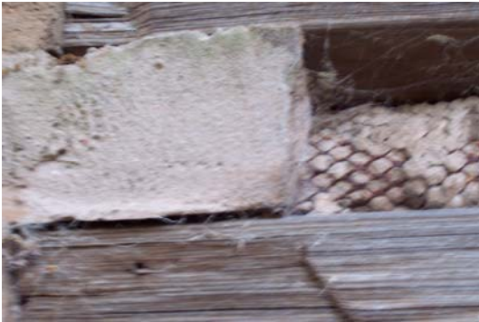
Figure 11.1 shows the concrete daubing used and the wire mesh chinking. This daubing is broken and as seen in figure 11.2 are typical. Many locations are void of daubing material and allow the light to enter the building. Daubing and Chinking require routine maintenance.
